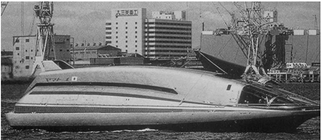
Figure 2.19 Yamato 1 : Experimental magnetohydrodynamic propulsion craft
