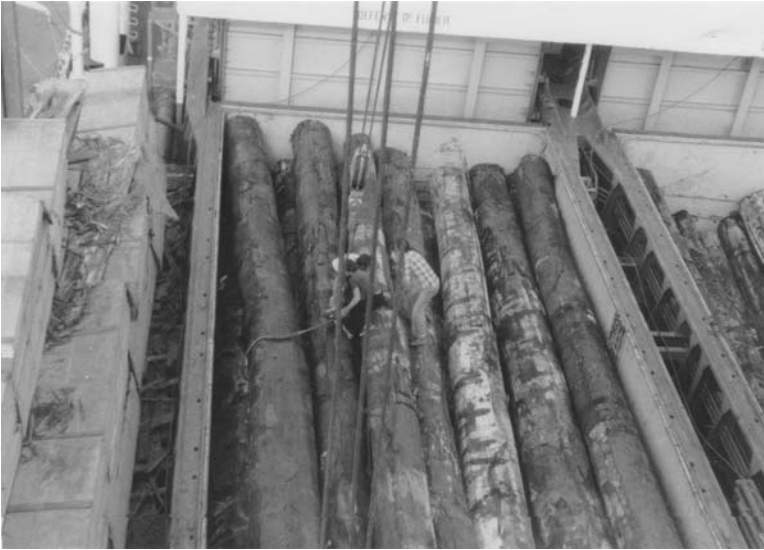
Plate 38. Logs being loaded upto the hatch coaming by use of wire snotters.
