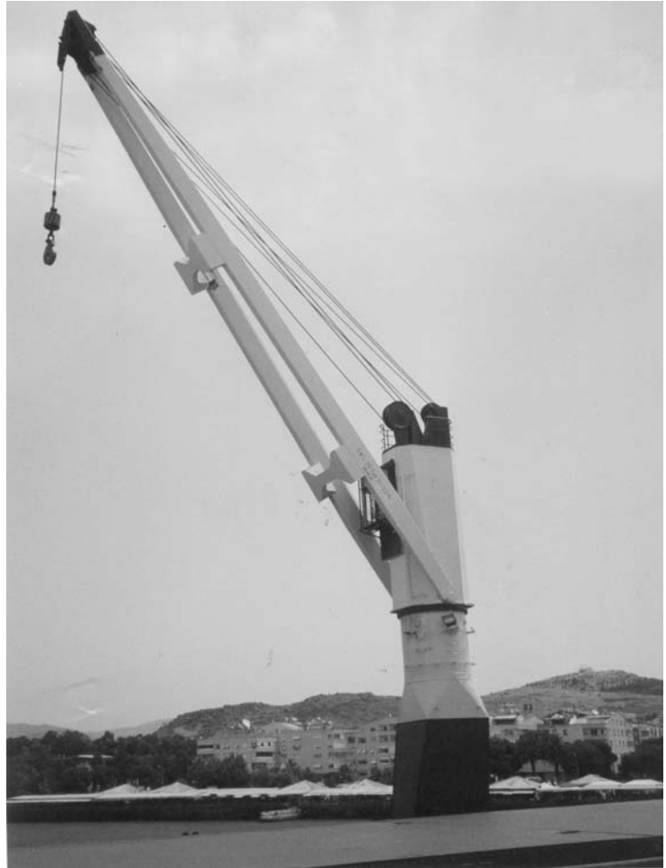
Plate 25. Deck crane with safe working load of 25 tonnes. On board the general cargo vessel 'Scandia Spirit'.
