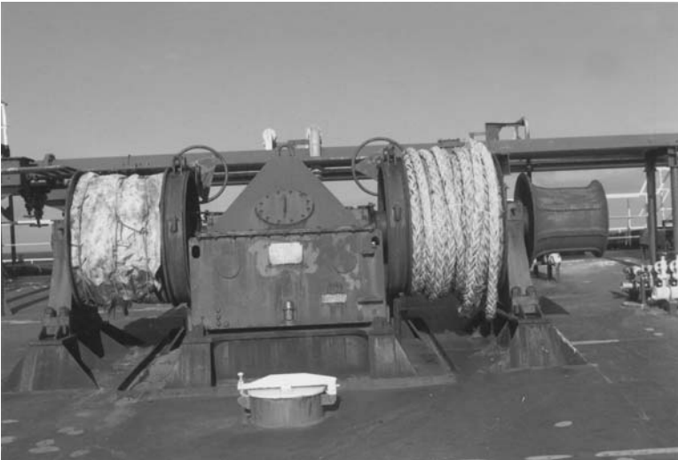
Plate 18. Tension mooring winch aboard a large tanker the winch barrels accommodate a multi-plaited mooring (synthetic) rope and a mooring wire (under canvas cover) an additional warping drum is seen at the end.
