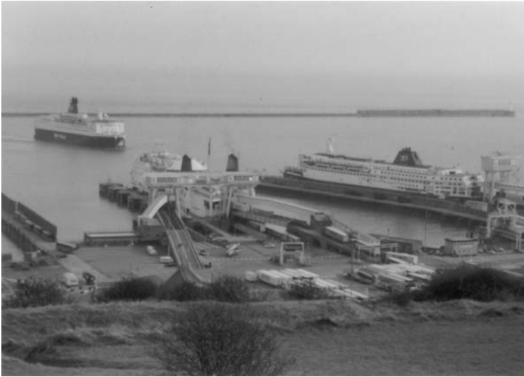
Plate 145. Ferry traffic in and around Dover Harbour. Heavy continuous traffic movement must be anticipated in such busy ports and harbours. Such vessels often require to turn off the berth to manoeuvre stern first in order to deploy vehicle ramps. They are also usually equipped with most of the modern ship handling hardware and as such sharp movements from bow and stern thruster units, twin CPP's and jet propulsion units must be expected by other ships in the vicinity.
