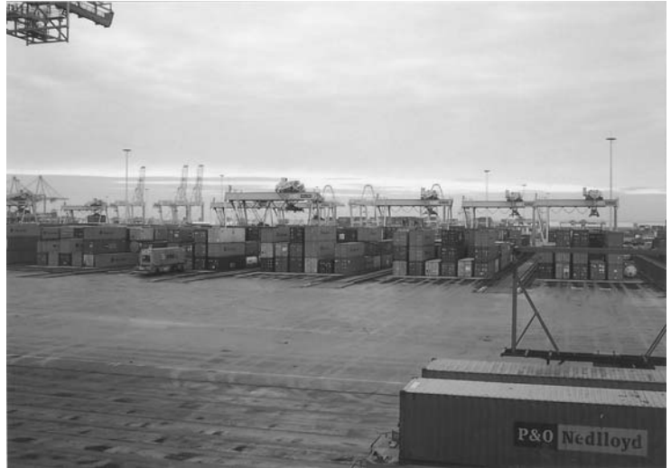
Plate 42. Shore side container terminal showing automatic stacking cranes in the background and the ship's loading gantry structure alongside.
