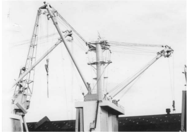
Plate 21. Heavy duty speed crane/derricks rigged for general cargo operations.
