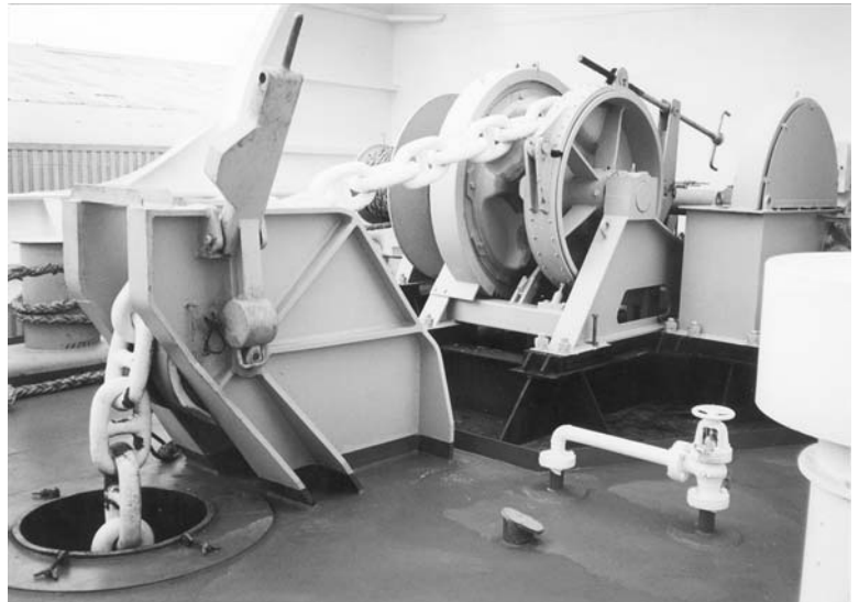
Plate 11. Arrangement of the starboard windlass aboard a modern RoPax ferry with split windlass operation.
