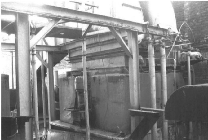
Figure 10-42. Ljungstrom air preheater.
