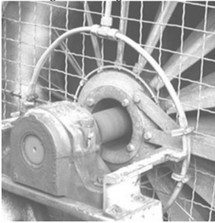
Figure 11-35. Fan inlet flow measuring ring.
