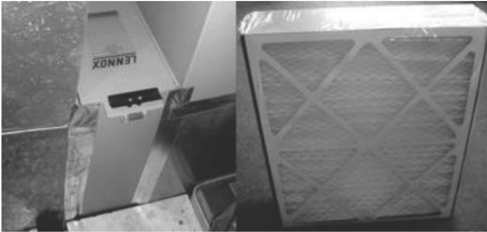
Figure 5-42. Home air filter box and filter.
