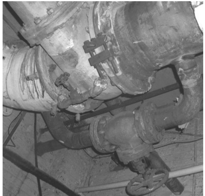
Figure 2-1. Warm up bypass valves.
