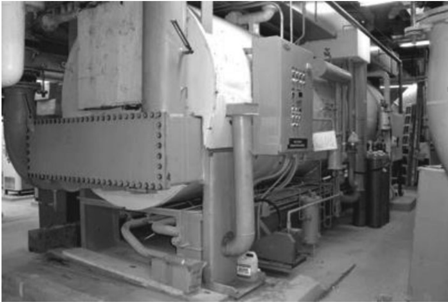
Figure 5-33. Absorption chiller.
