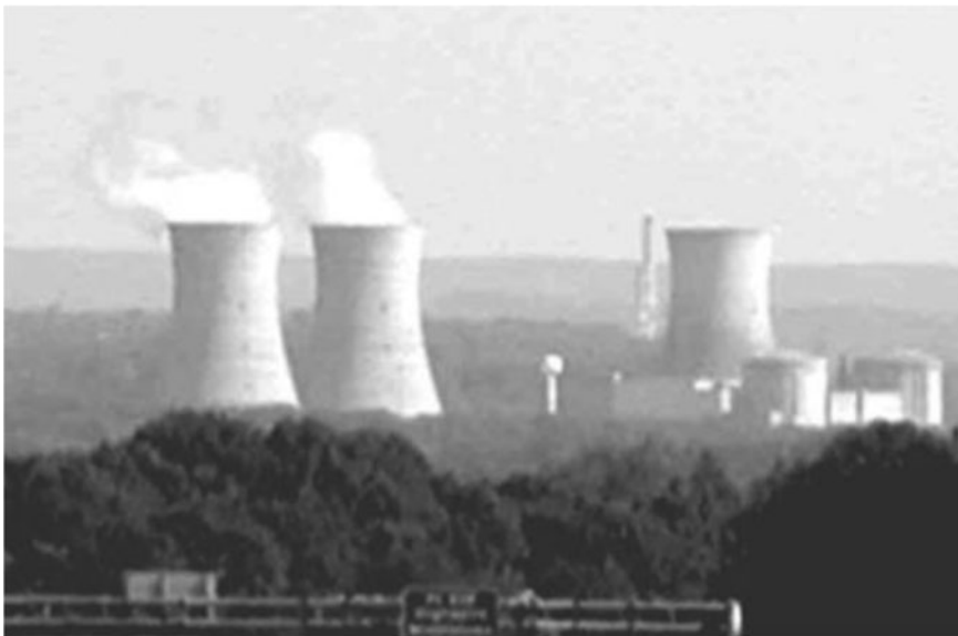
Figure 5-39. Hyperbolic Cooling Tower in a Power Plant
