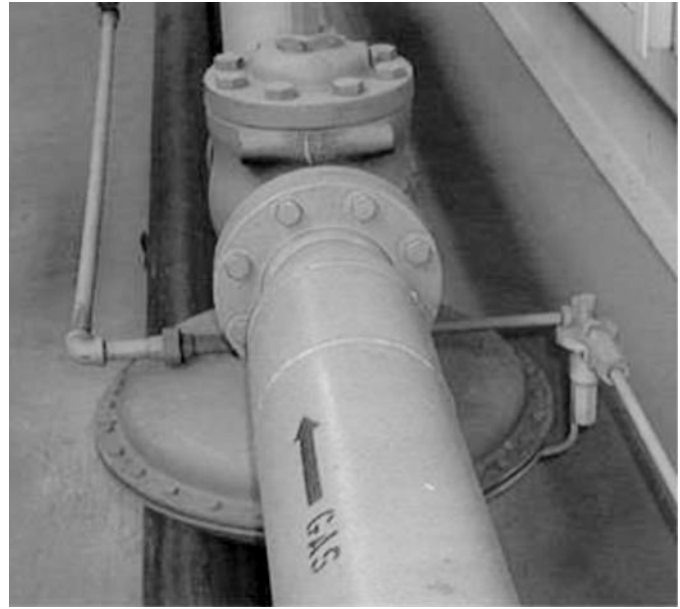
Figure 11-17. Piloted gas pressure regulator.
