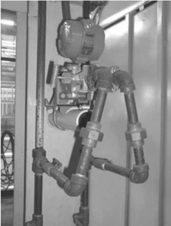
Figure 11-40. Proper transmitter installation.
