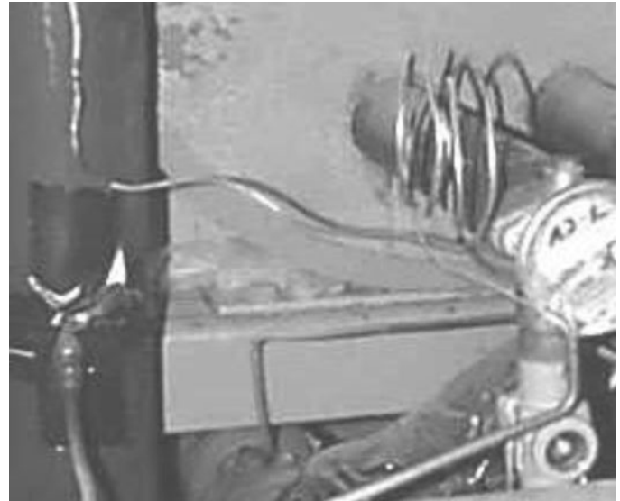
Figure 5-25. TXV installation.
