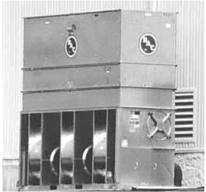
Figure 5-36. Blow-thru cooling tower.
