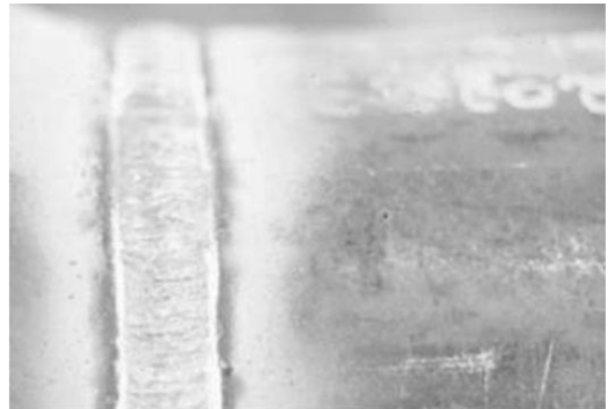
Figure 6-21. Cover pass of completed weld.
