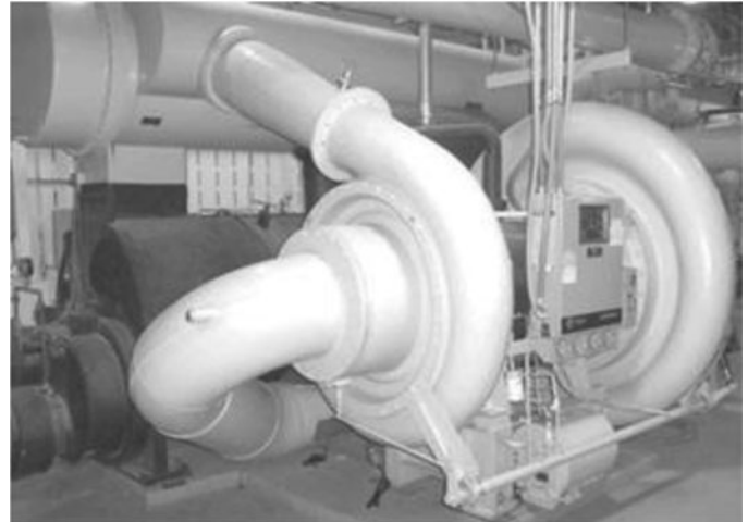
Figure 5-32. Centrifugal chiller with two-stage compressor.
