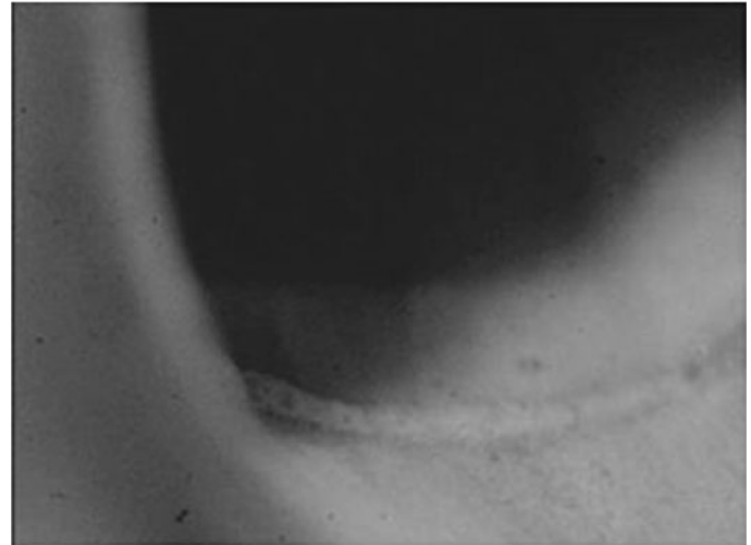
Figure 6-16. View inside of root weld.
