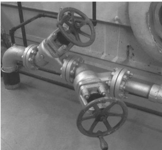
Figure 2-6. Seatless blow off valves.
