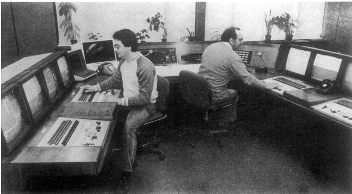
Figure 48.28 A surface control room
