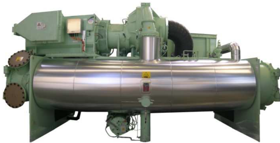
Figure 39: Centrifugal chiller that can use R513A instead of R134a
