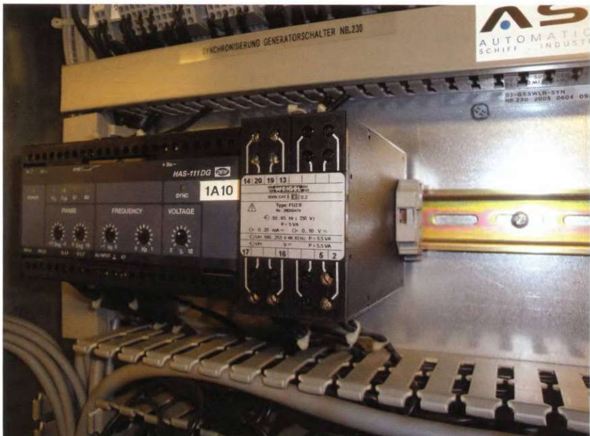
Figure 3.15b - Synchronising unit
